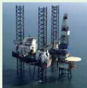
In 7 months Wintershall dismantled the K10 V platform and after refurbishment installed the L5C platform for the extraction of approx. 4.3 bln m³ of Natural gas. The reuse of a platform can both be environmental friendly and economical.
