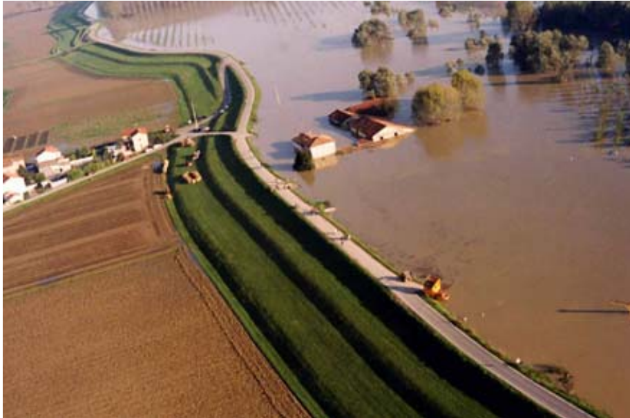
Figuur 10-6 Main levee along the river Po, in the vicinity of the town of Agoiolo, with a house in the floodplain. Agricultural activities such as fields and young plantation trees are also visible.
