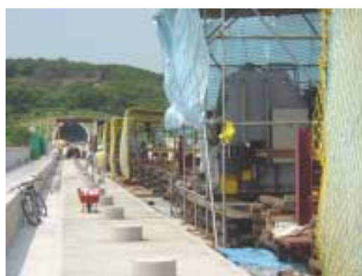
THSRC Construction showing walkway extreme left
