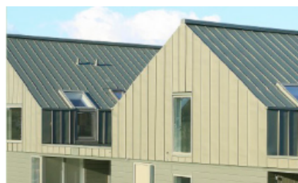
houtstructuren dmv felsbanen
