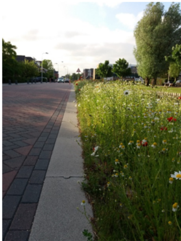
Figuur 7 Afwatering in berm, Aardamseweg Ter Aar
