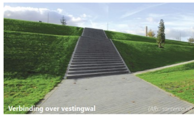
Verbinding over vestingwal (Afb. - santenco.nl)
