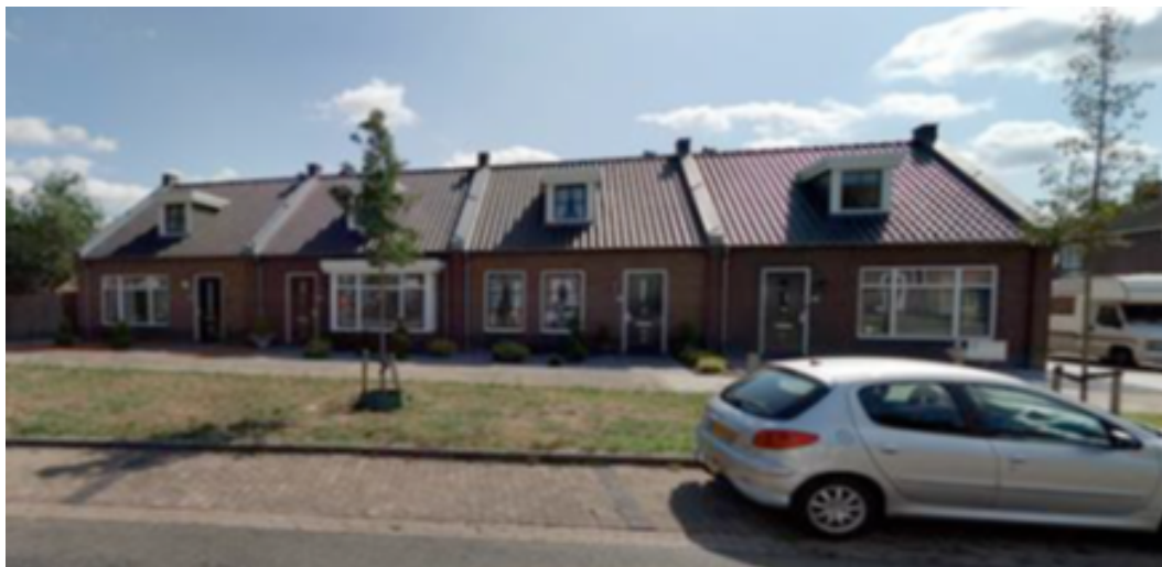
Multifunctionele woningen Destion in Nieuw Bergen
