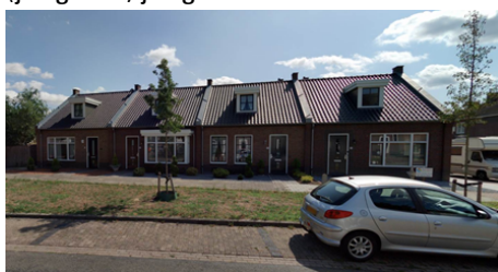
Multifunctionele woningen Destion in Nieuw Bergen
