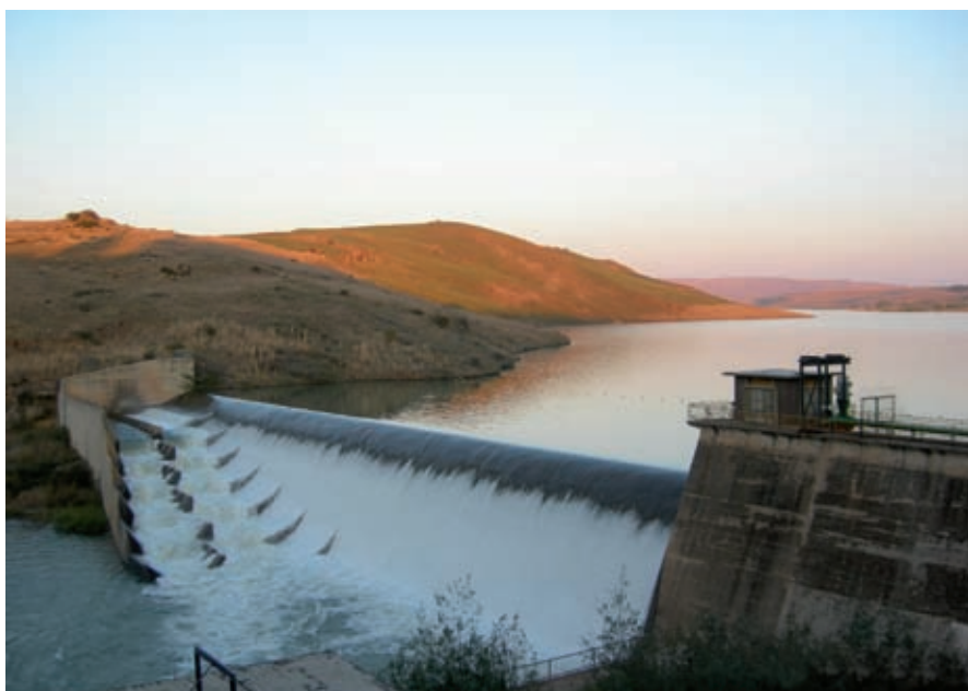
Hydropower project in South Africa (2006)
