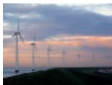
page 33 Dronten Number of turbines: 28 Rotordiameter: 43 m Hubhight: 50 m
