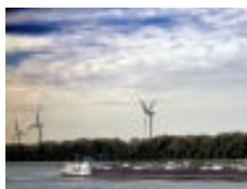
page 7 Volkerak dike Number of turbines: 4 Rotordiameter: 44 Hubhight: 55 m
