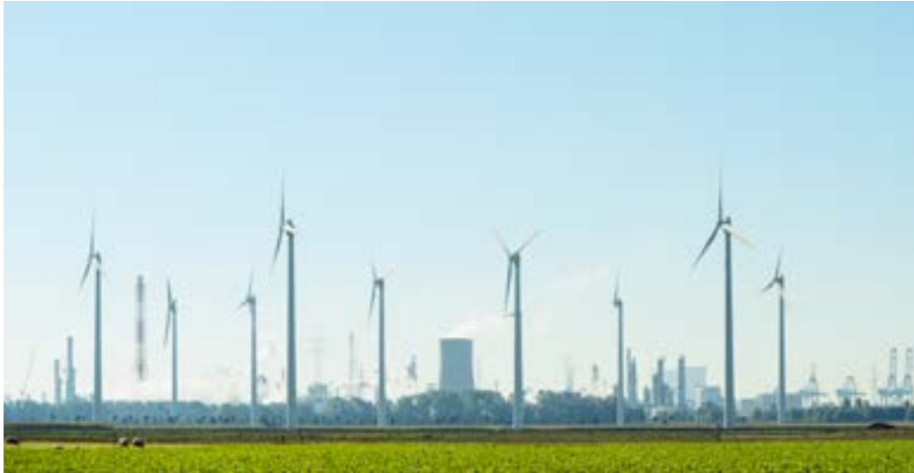
Windpark Rilland in Zeeland.
