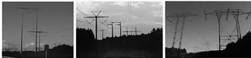
Figure 6.30 HVDC line configurations: (a) Brazil 600 kV tower; (b) Rihand-Delhi 500 kV HVDC; (c) Quebec-New England HVDC interconnection \pm 450 kV line.
