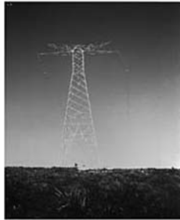
Photo 11 Self-supporting 600 kV tower
