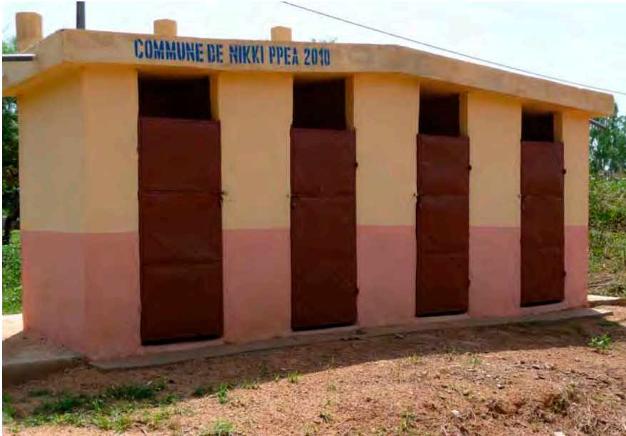
Latrines in institution
