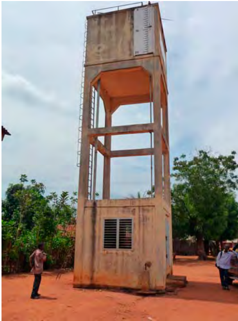
Water tower small piped water supply system
