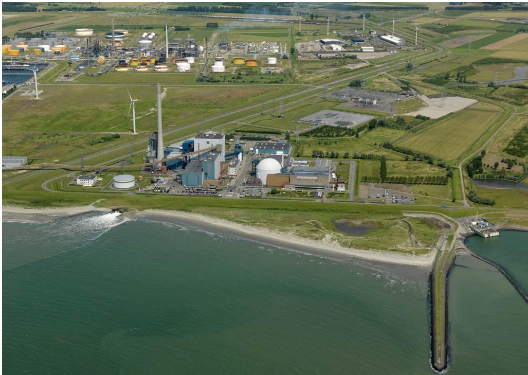
Figure 1.2 An aerial photograph of the Borssele site
