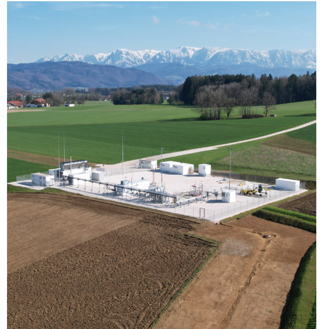
RAG underground hydrogen storage facility, Rubensdorf , Oostenrijk
