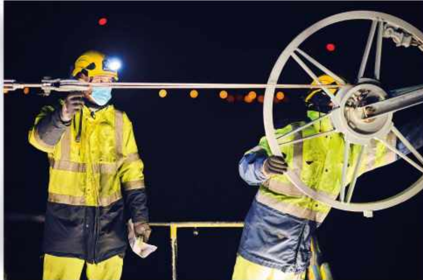
Electrification works on the line between Mol and Hamont Photo: Infrabel – Benjamin Brolet
