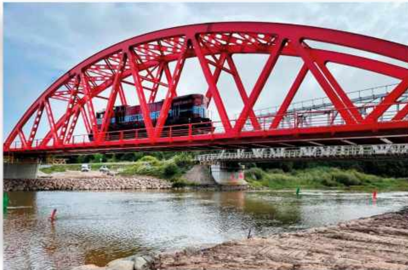
Railway bridge across the river Emajõgi near Tartu Photo: Eesti Raudtee AS
