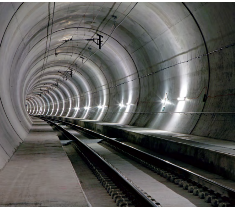
Inside the Lötschberg base tunnel.
