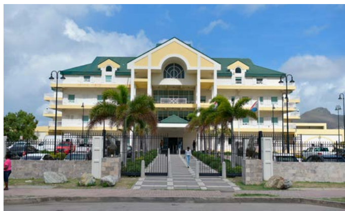
Photo 4: Government Administration Building
