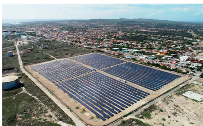
Renewable Energy, wind and solar, infrastructure in Aruba.
